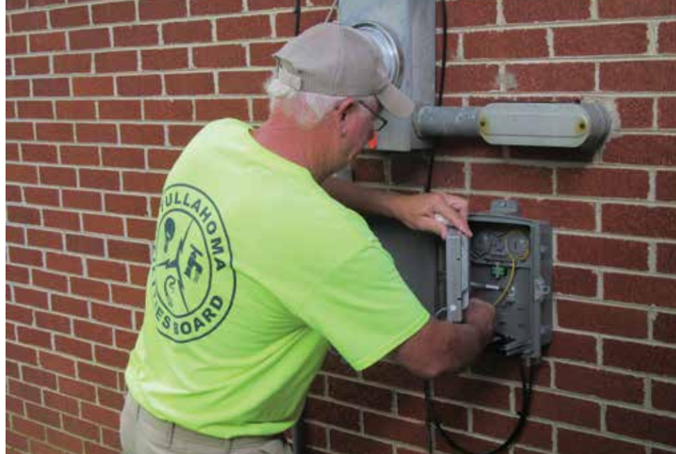
LightTUBE Installer Robert Overman assists in a residential installation.
