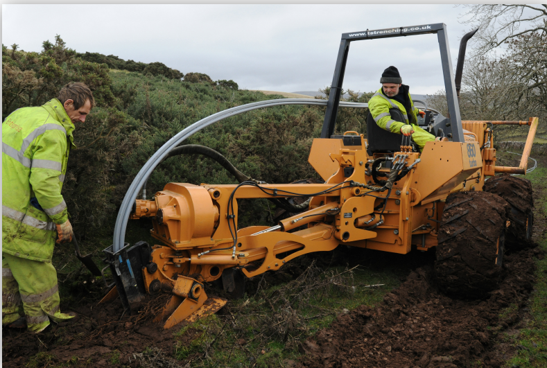
Fiber installation. (Photo credit: btphotosbduk, licensed through Creative Commons)
