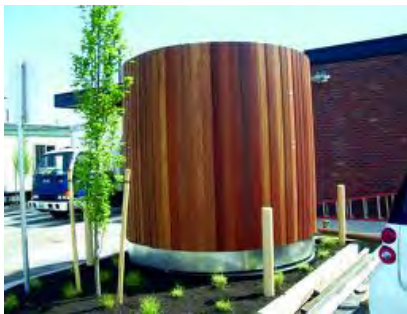
Image 5.4 (Left): Rain Water Cistern
