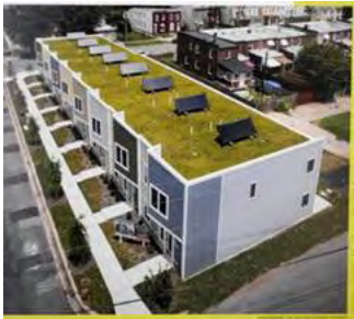
Image 5.11: Residential area with Green Roofs and Solar Panels
