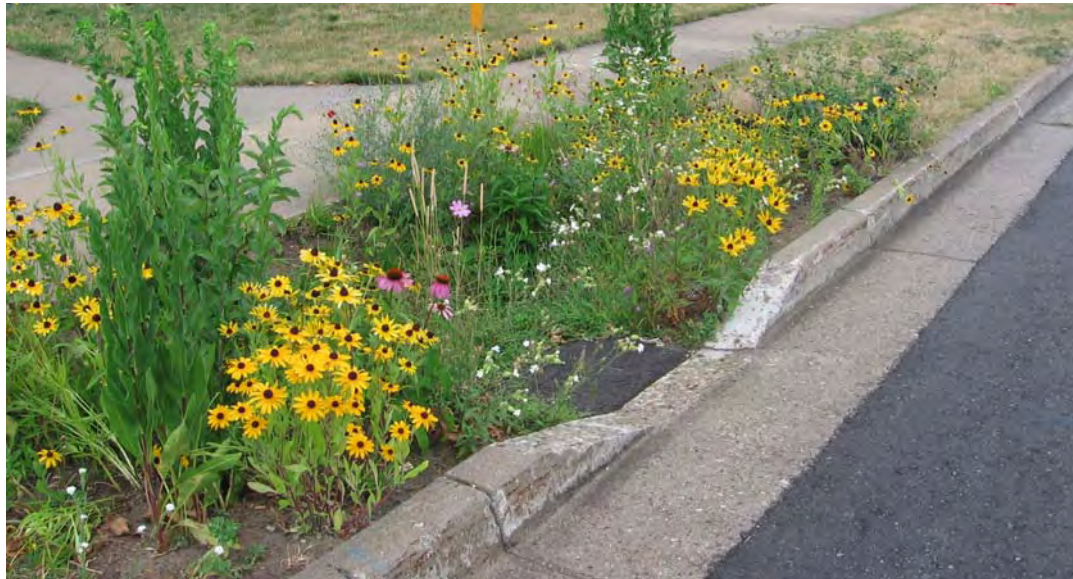
Image 4.11: Curb-cut into bio-retention area.
