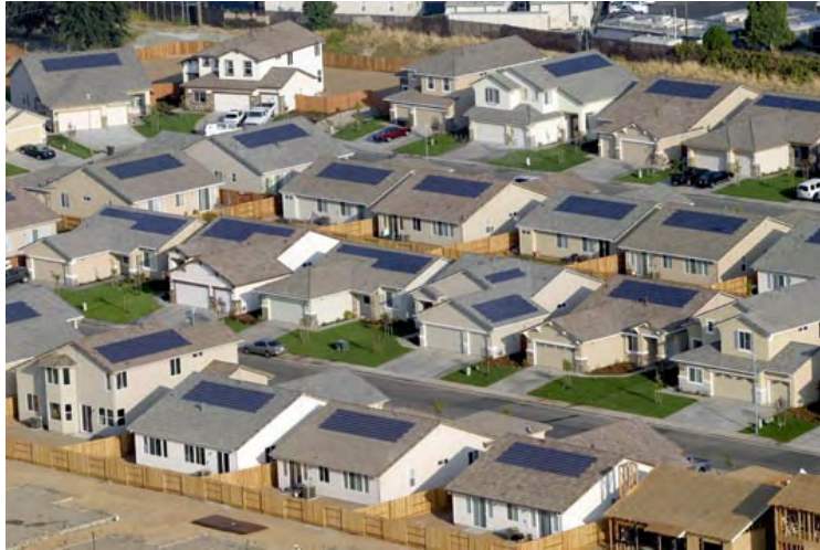
Image 5.6: Solar roof tops.
