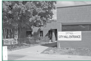
While construction is underway, the entrance to City Hall is located on the south side of the building with parking available in the lot between City Hall and Fire Headquarters. Thanks for your patience and cooperation during the project!
